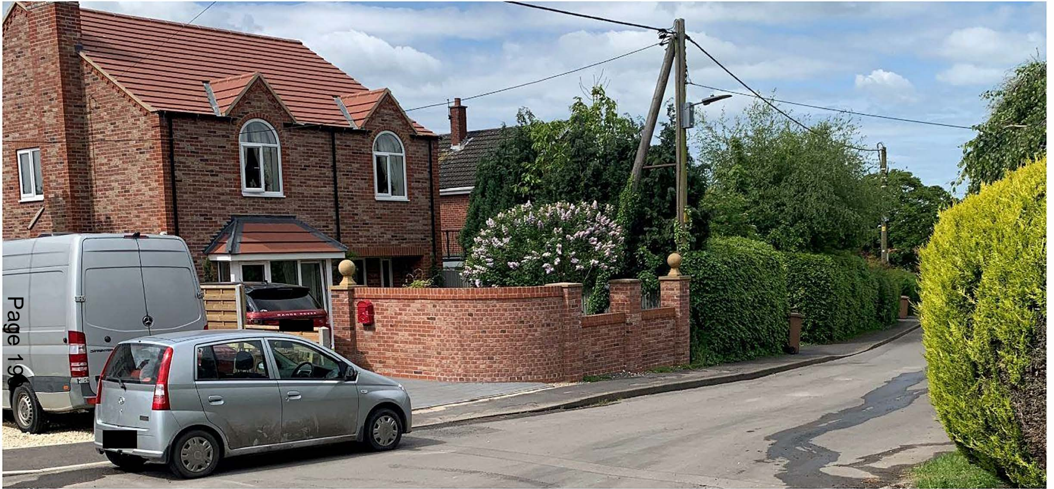
PA/2023/67 Photograph of wall in situ
